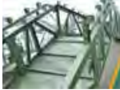
Truss/Painted Angle Steel
