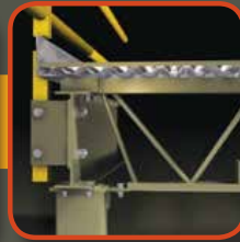
BEAM & BAR JOIST
